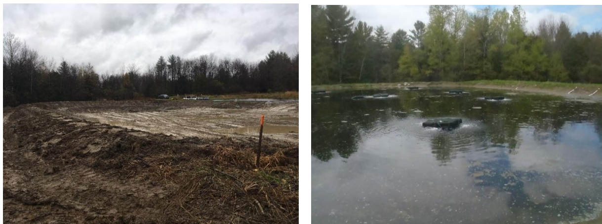
Figure 9. Lake Carmi State Park zero discharge wastewater treatment system under construction (left) and constructed with operational aeration “islands” (right).
