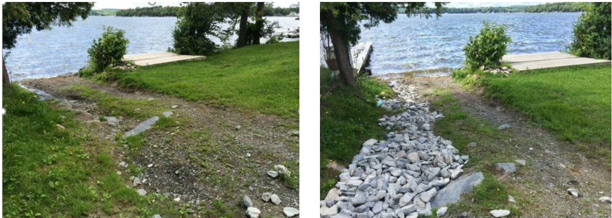
Figure 7. Before (left) and after (right) stabilization of an eroding lakeshore access path to Lake Carmi, completed by the Franklin Watershed Committee as part of the Lake Wise Program with funding from DEC’s Clean Water Initiative Program.
