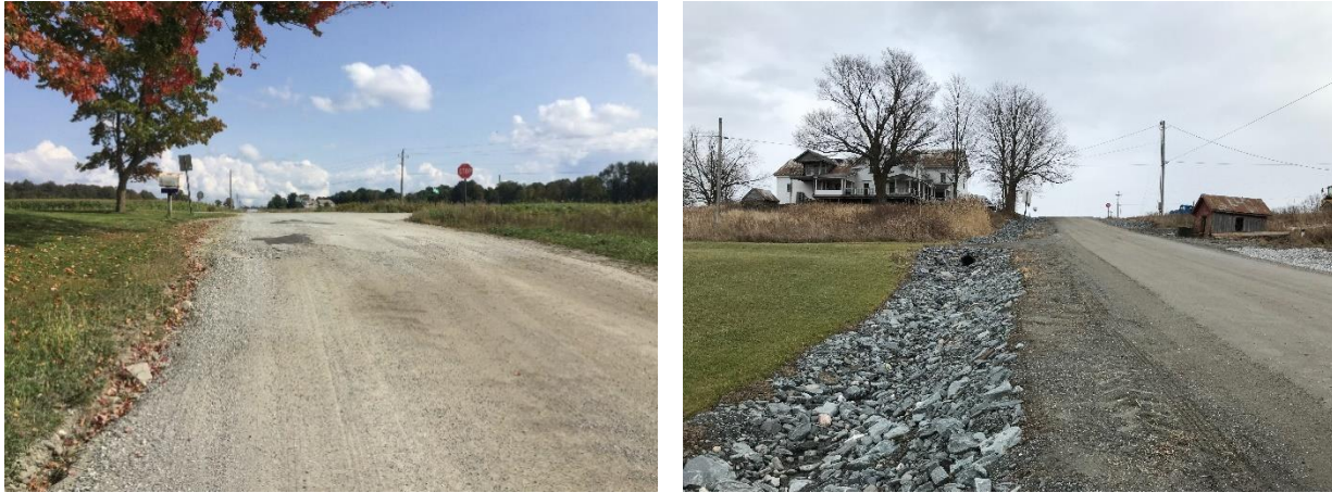
Figure 8. Before (left) and after (right) installation of stone-lined drainage ditch and road drainage culvert along Dewing Road by the Town of Franklin, in partnership with Northwest Regional Planning Commission funded through the Municipal Roads Grants-in-Aid Program.
